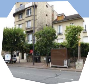
Melun (77), Ex-RN6 Station Oper@Ex
