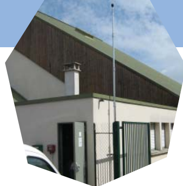
Villabé (91) -A6 Station Oper@Ex
